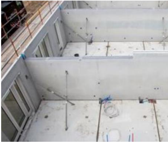
Figure 3. Placing of prefabricated concrete elements.
