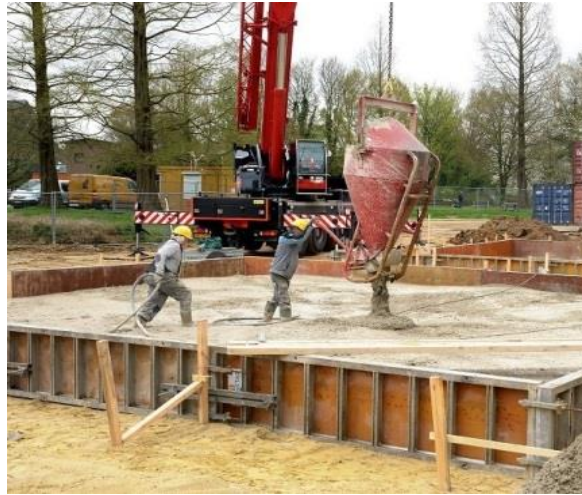
Figure 4. On-site pouring of recycled concrete.
