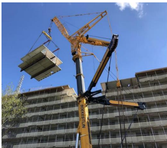
Figure 1. Complete compartment being hoisted out.
