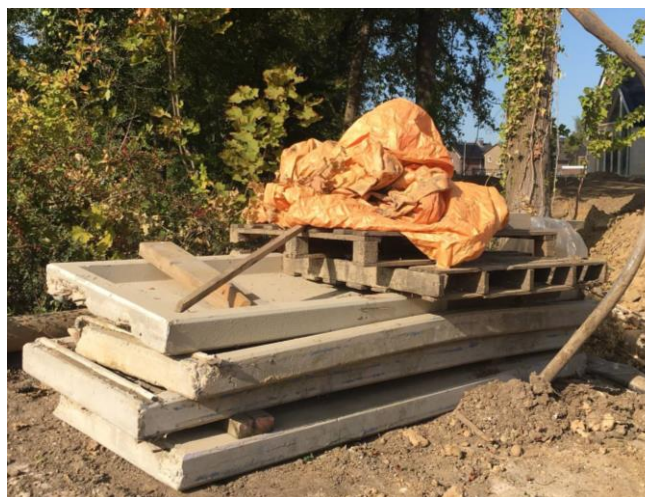
Figure 2. Damaged slabs intended for reuse.
