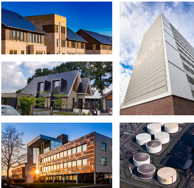
Fig. 2. Examples of realised BIPV projects in the Netherlands. Top-left: full solar roof (source: Exasun); top-right: solar facade (source: Zigzagsolar); middle-left: solar roof tiles (source: Solinso); bottom-left: coloured solar facade (source: Solarix-solar); bottom-right: solar roof membrane (source: HyET Solar).
